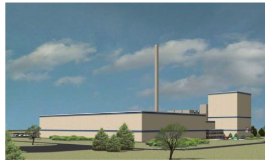
Figure 23. Fibrowatt plant, Benson, MN
